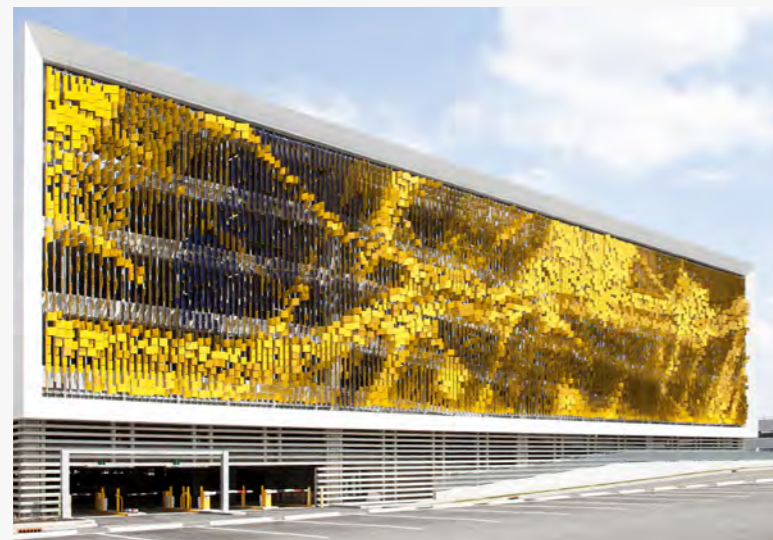
STATIC DYNAMIC FACADE CREATED BY BENT BLADES ESKENAZI HOSPITAL PARKING STRUCTURE
