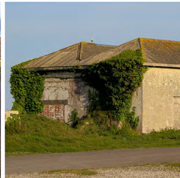
OLD INCLINE ENGINE HOUSE, INCLINE ROAD
