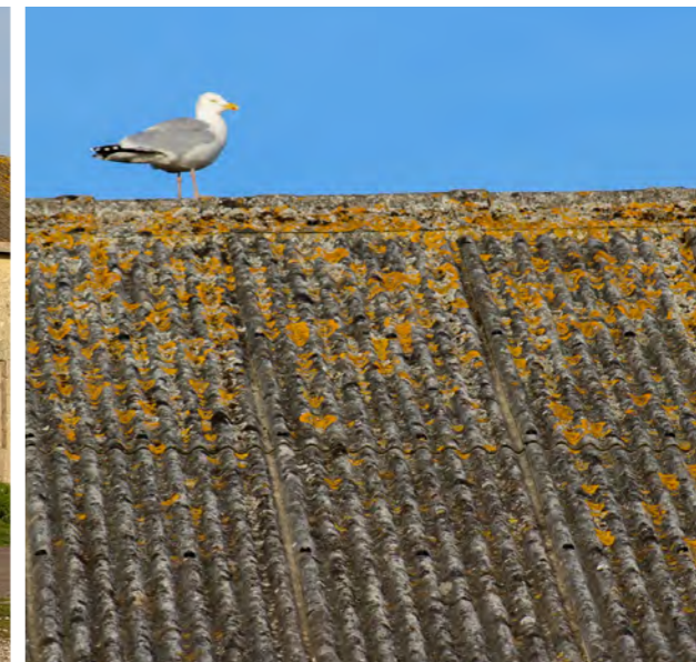
OLD INCLINE ENGINE HOUSE - SINUSOIDAL ROOF SHEETING WITH MOSS AND LICHEN
