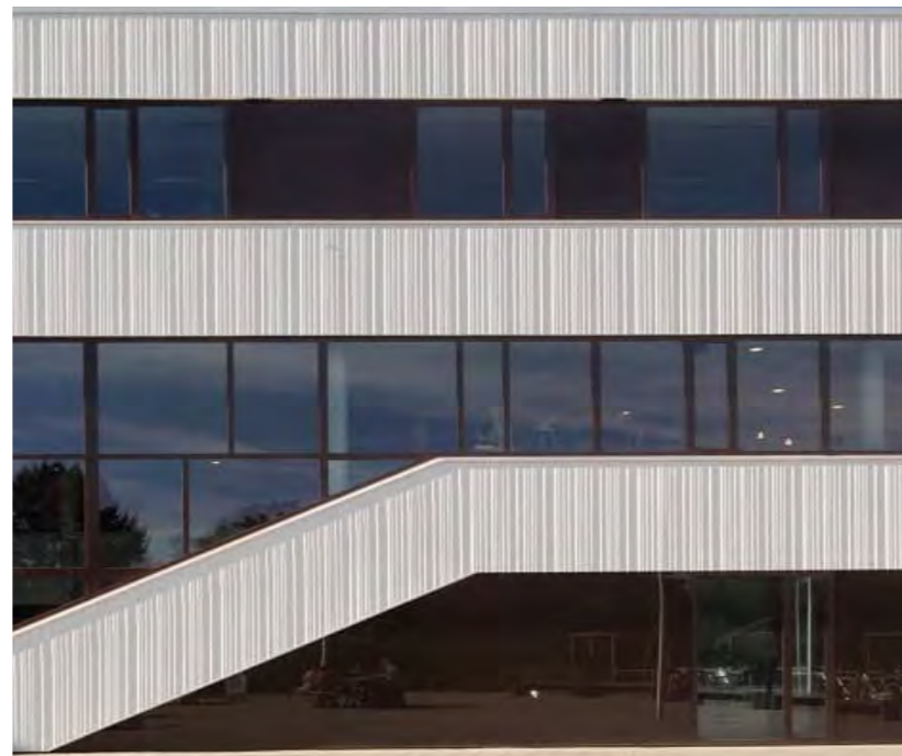
SUBTLE VERTICAL FEATURES CREATING DEPTH AND RELIEF TO THE FACADE PRECEDENT PROJECT
